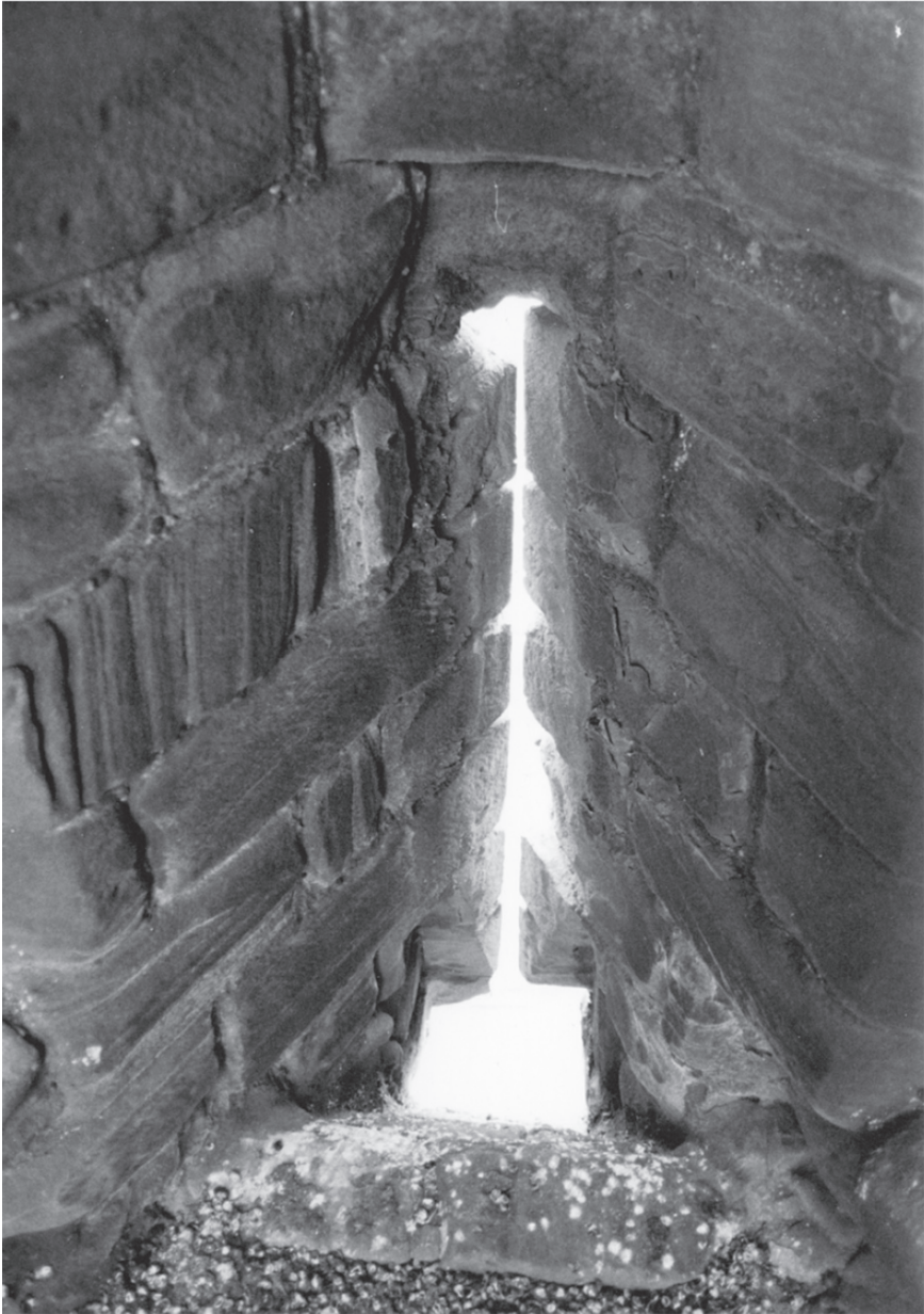
Figure II.12.7 Kenilworth (GB). Interior of an embrasure in the Great Tower, with an hypertrophic square hole, behind the also hypertrophic fishtail base (see Figure 12.5). © Castle Studies Group, photo R.K. Morris
