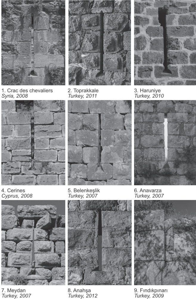
Figure II.12.3 Synoptic view of different enlarged bases. © Maxime Goepp
